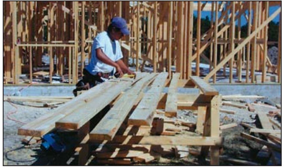
Eusevio Rios, of Lakeridge Custom Homes, marks rafters for the Longo residence in Dripping Springs.
