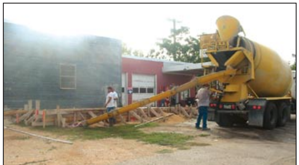
Crew with Alpha Concrete pouring a slab in downtown Liberty Hill.
